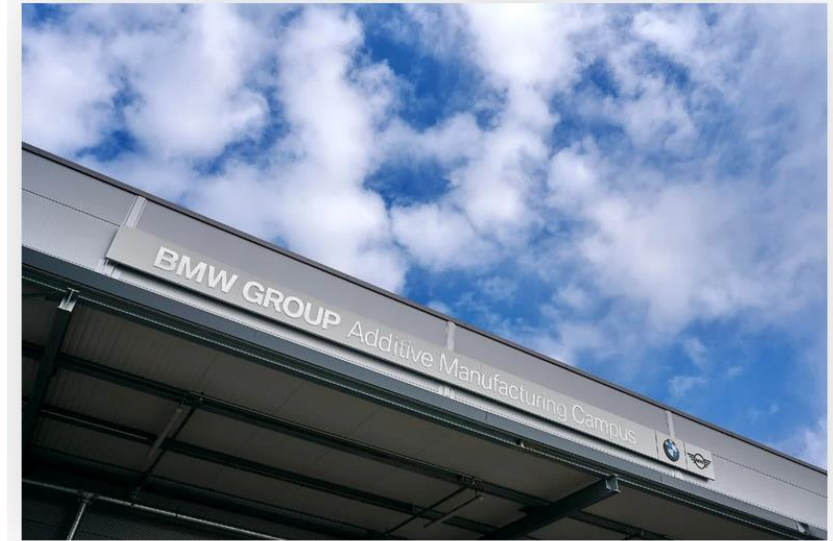
The new Additive Manufacturing Campus will have a huge influence on future BMW Group production. (Source: BMW)
